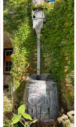
Decorative cistern at the base of an ornamental leader
