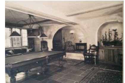
^^ Found opportunities: 1 st floor northwest corner space with screened-in porch as an outdoor conference room
